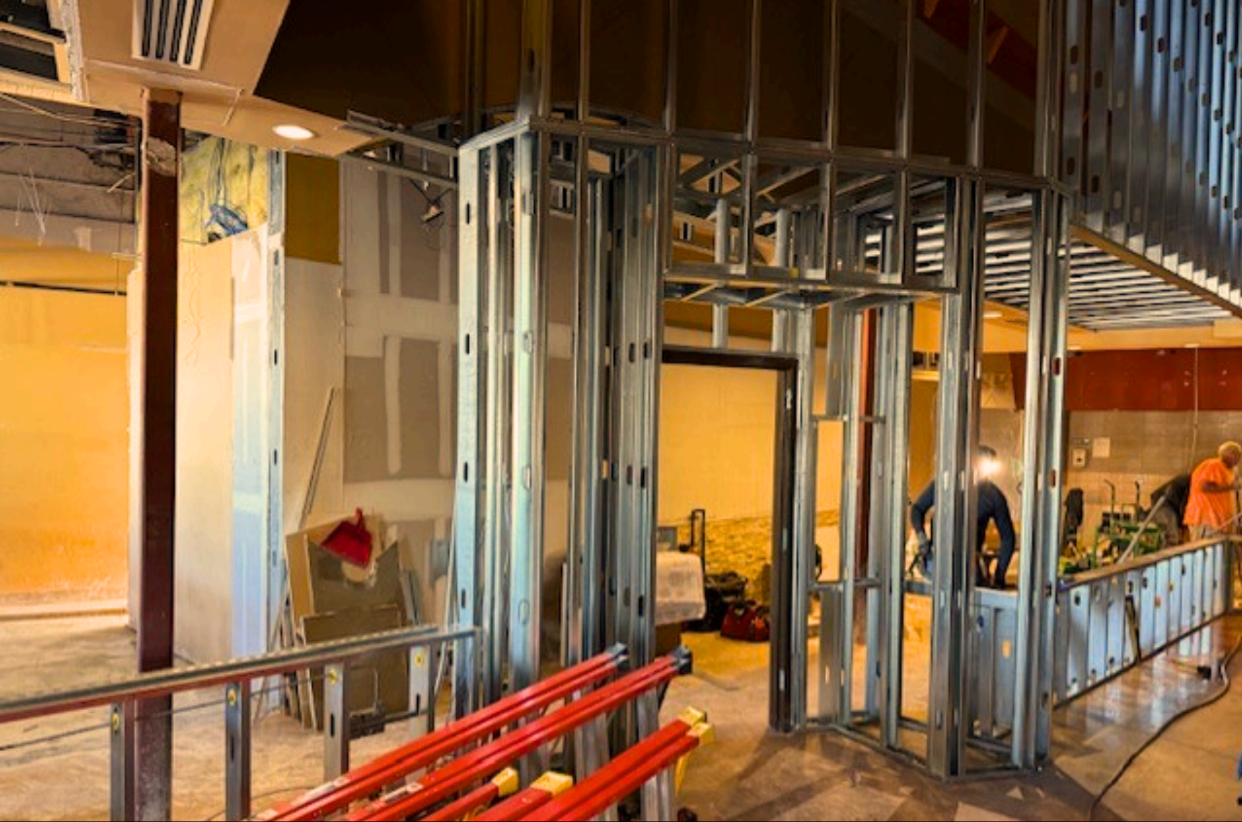
The construction process is underway on renovating the concessions area at EPIC's Deltona, FL flagship location.
